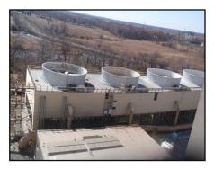
wood replacement on two (2) complete cells during a defined 2015 outage. As an option, EvapTech suggested that while there would be a "complete" outage, replace all structure below the water level in all six (6) cells. That additional scope (in green) was well received and fully executed during the 2015 outage. (Cells 1 & 2 completed in 2015, Cells 3 & 4 slated for 2017 and Cells 5 & 6 for 2016)
