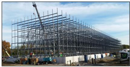
Since the plants were identical to one another, both cooling towers were purchased under a single contract. This allowed EvapTech to engineer and design one tower for both sites and purchase the components in bulk, creating significant cost savings that were passed on to the customer. Each tower is 7 cells with a total water flow in excess of 100,000 GPM.
