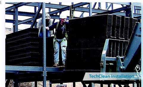
Fire Safety – TechClean PVC film fill packs reduce the risk of fire propagation.
