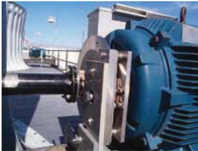
The Addax Cooling Tower Brake is a mechanical, manually-actuated caliper disc brake for stopping, holding and locking out cooling tower fans. It easily adapts to the motor hub of the Addax Composite Coupling.
