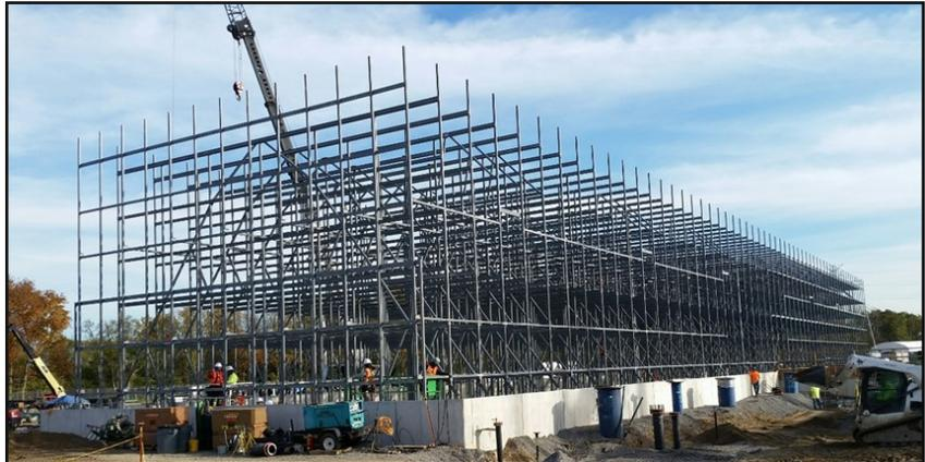
Since the plants were identical to one another, both cooling towers were purchased under a single contract. This allowed EvapTech to engineer and design one tower for both sites and purchase the components in bulk, creating significant cost savings that were passed on to the customer. Each tower is 7 cells with a total water flow in excess of 100,000 GPM.
