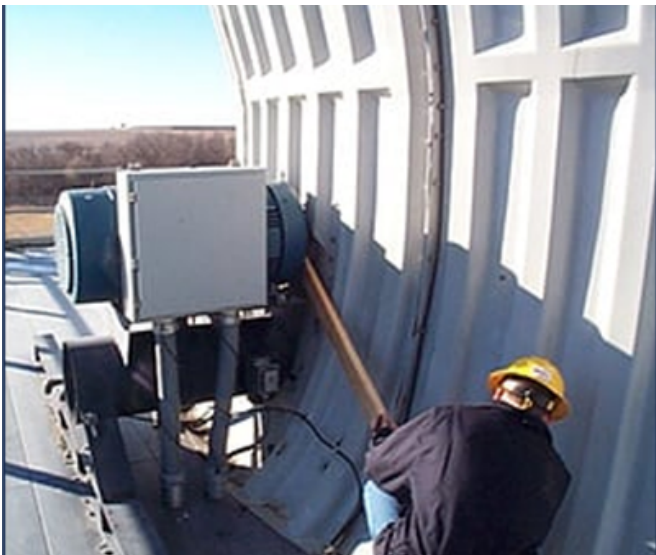
Fig 2. Example using a board to arrest rotation
