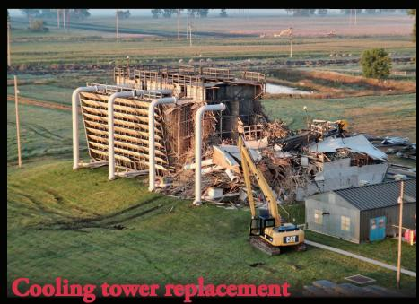
**Above** An excavator brings down the 50-plus-year-old redwood cooling tower at Wisdom Station, Spencer. A new fiberglass tower will be constructed this fall.
